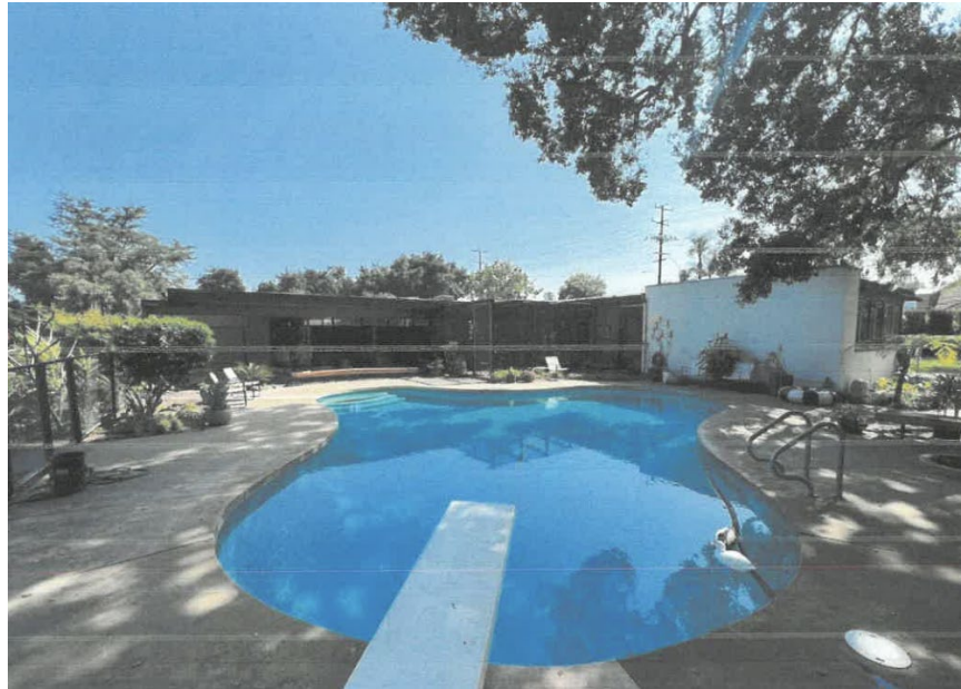
Figure 5 - Northeast elevation of the home, walls will be repainted and/or re-stuccoed
